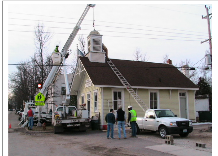
“Old City Hall” Renovation Underway
